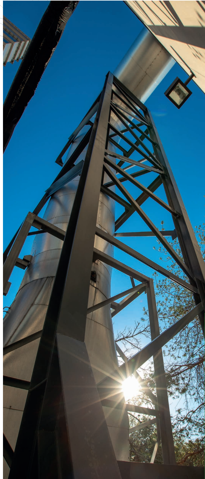
Quad's manufacturing facilities are equipped with advanced regenerative thermal oxidizers (RTOs) — pollution control devices that combust and decompose VOCs into CO 2 and water vapor.
